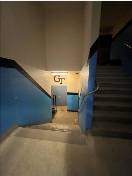
MEZZANINE TO FIRST FLOOR, NORTH
